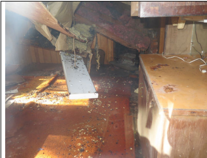
ABOVE: View of the interior of the cabin looking from deck through a window. (9536)
