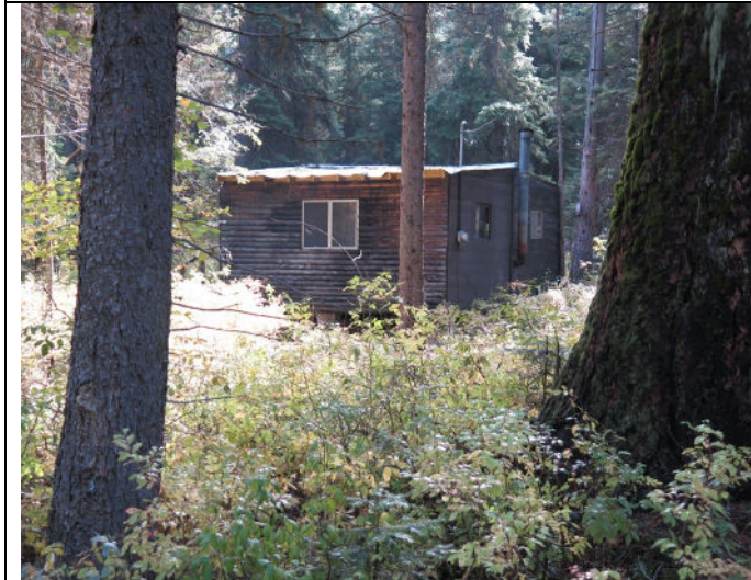
ABOVE: Close-up of the west and south (right) elevations of the existing cabin. (9523)
