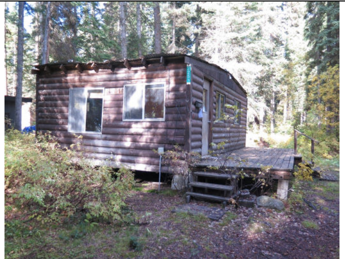
ABOVE: Close-up of the existing cabin showing the north (right) and east elevations. (9534)
