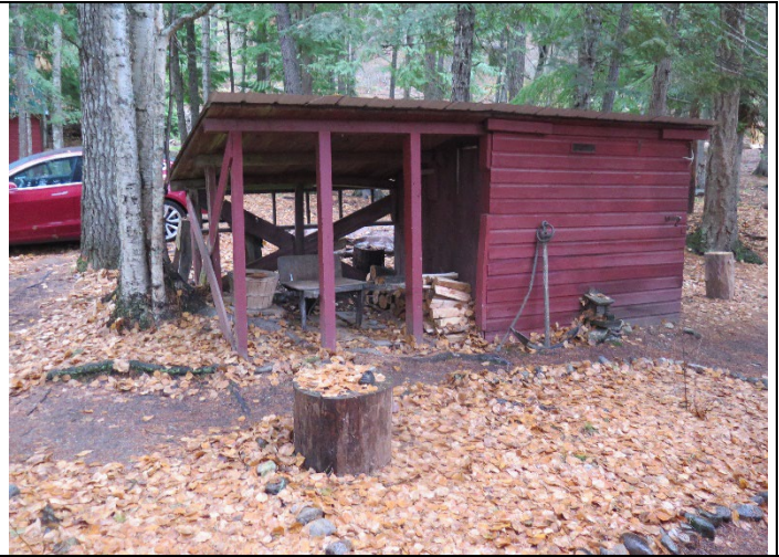
ABOVE: Small firewood/storage building. (4985)
