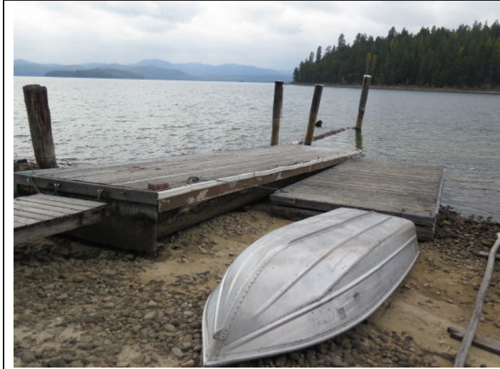
ABOVE: Close-up of the dock improvements. (1129)
