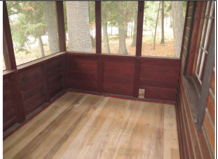
ABOVE: North side of Screened-in porch. (1153)
