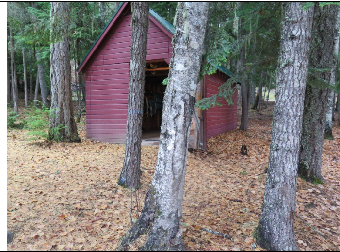
ABOVE: View of the detached garage. (4989)
