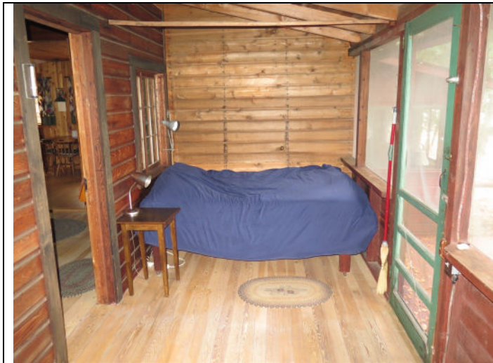
ABOVE: Another view of the screened-in porch to south side of area that is used as a sleeping area. (1154)
